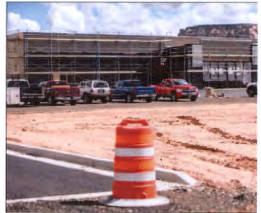
A new supermarket is under construction in Zuni Thursday.
